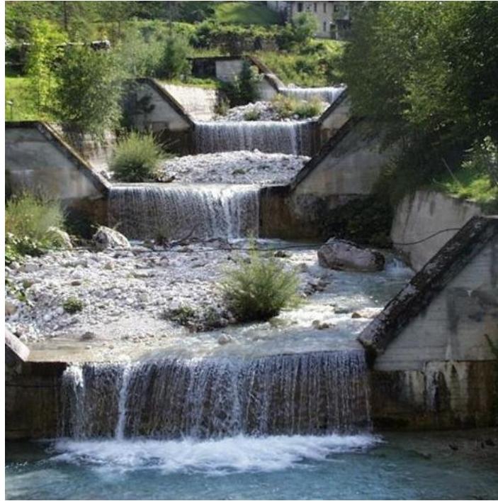
Figure 16. Check dams in Pramper River, Italy (Comiti et al., 2013)
